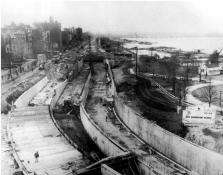
Figure 4.1 – This 1951 view shows construction of the Storrow Drive Tunnel with fill from the tunnel used to create additional parkland. (from Mapping Boston)
